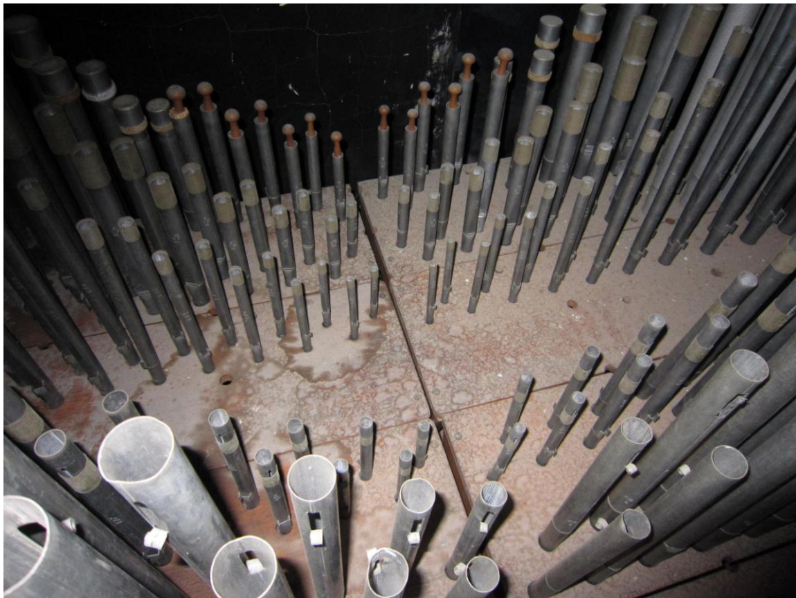
The water damage to the Great soundboard of the Masonic Temple Brisbane.
